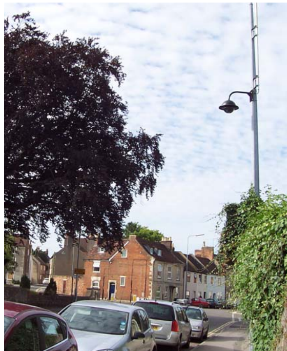
New camera installed at Portway
